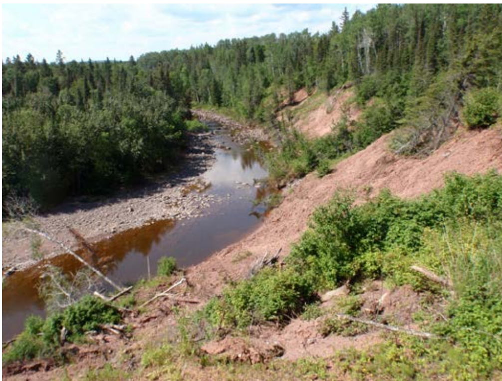
Photo 5-1 Pre project view of the project site July 10, 2012. Slumping and mass wasting of the large clay bank was contributing significant sediment loads to the Knife River.
