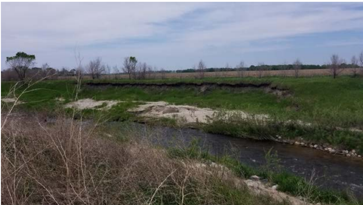
Photo 15-6 Downstream view of riffle #13. Note the erosion on the bare slopes of the far bank. Photo taken by Ed Matthiesen during site visit (6/4/2019).
