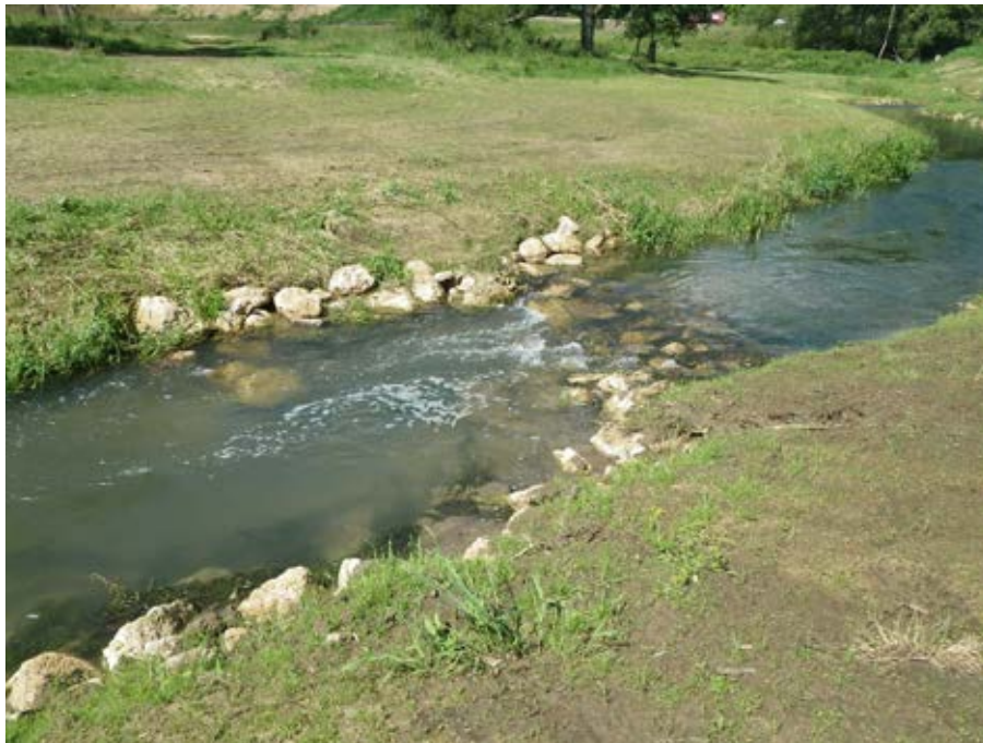
Photo 22-8. Example of a vortex weir installed in 2011. It is used to hold the grade of the upstream pool and create a plunge pool on the downstream end. Photo taken August 2011 and provided by MN DNR.
