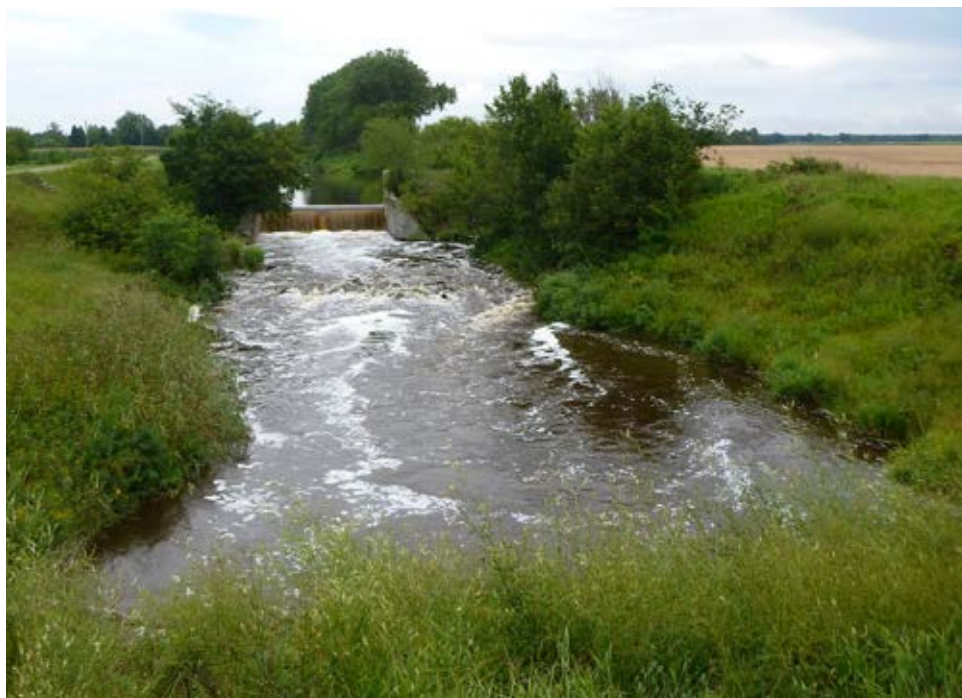
Photo 16-1 Drop structure 4 prior to modification. Photo provided by project partners (taken 8/16/2016).
