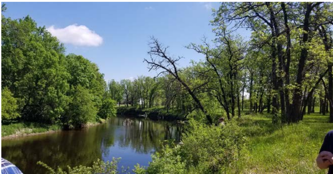
Photo 11-1 Upstream view of stream barbs 3 and 4 with some bare slopes downstream and trees leaning over the river. It is recommended to install live stakes on the bare slopes, provide a buffer to the top of the bank, and remove the leaning trees and limbs. Photo taken by Ed Matthiesen during site visit (6/5/2019).
