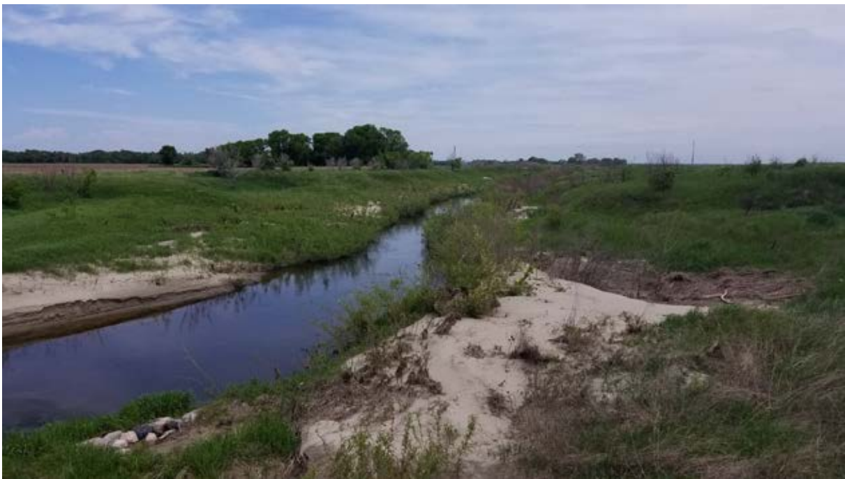
Photo 15-4 Upstream view of riffle #13. Note erosion on the bare bank (left). An observed opportunity for improvement is to add sandbar willow. Photo taken by Ed Matthiesen during site visit (6/4/2019).
