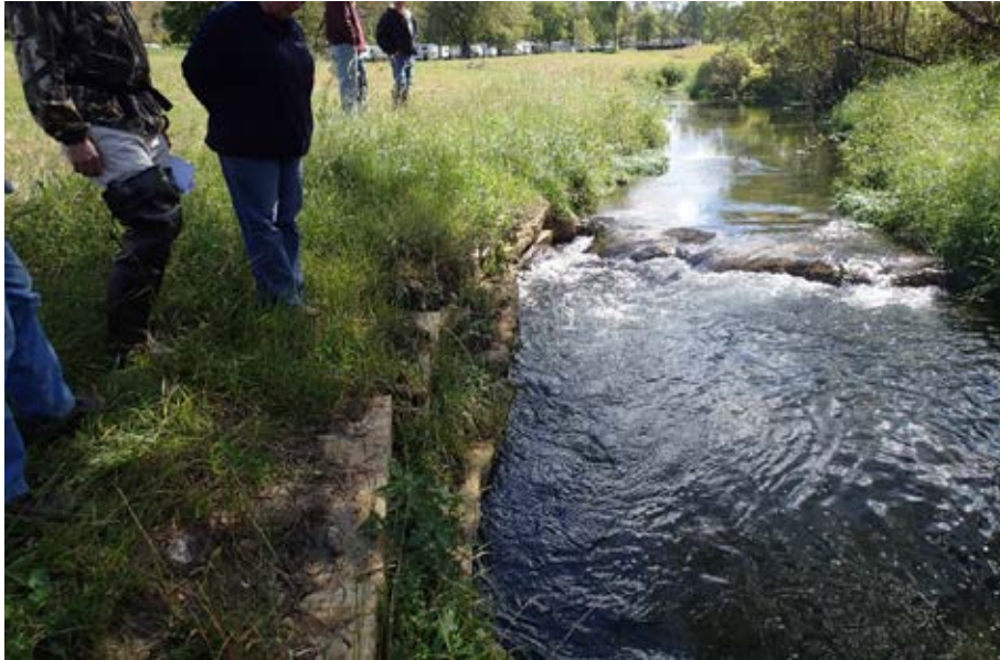
Photo 33-5 Regraded slope, Rock deflector and Rock weir. Site visit 09/18/2012.
