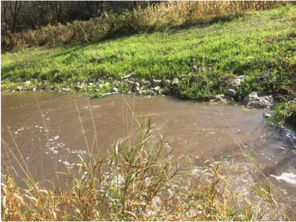
Photo 19-3 Additional rock added in 2019. Photo taken 10/21/2019 by Anna Varian.
