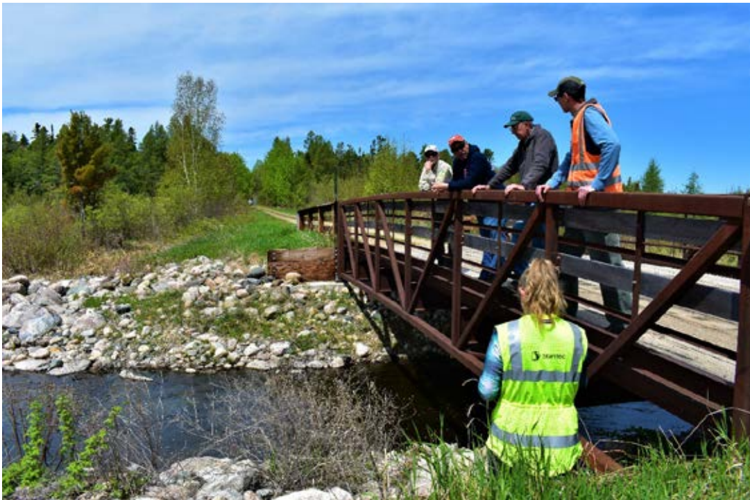
Photo 23-6 Project partners discussing the outcomes of the work on the bridge installed over the riffles to maintain access to the snowmobile trail that previously ran over the dam, taken 5/28/2019.
