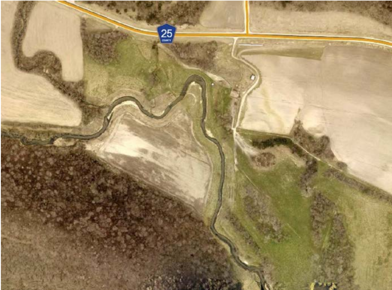
Photo 29-1 Aerial of the project site from 2016, 5 years after construction. Aerial imagery provided by Winona County, Minnesota.
