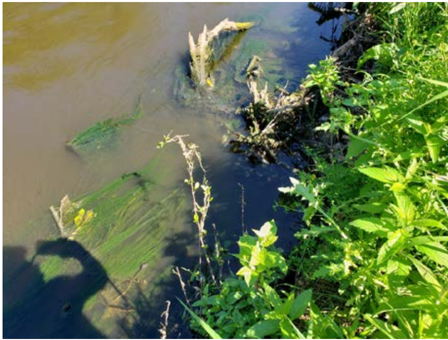
Photo 30-7. Example of the toewood bench on the treatment bank. Typically in the toewood installations the majority of the rootwads, logs, and other coarse woody material remains submerged to prevent rotting, reduce shear stress against the bank, and provide aquatic habitat for fish and invertebrates. (Photo taken 6/26/19 by Mark Pranckus, Cardno).
