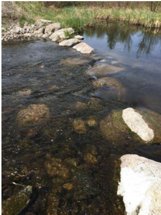
Photo 23-5 View of topmost weir and spaces between weir for fish passage, taken 5/28/2019.
