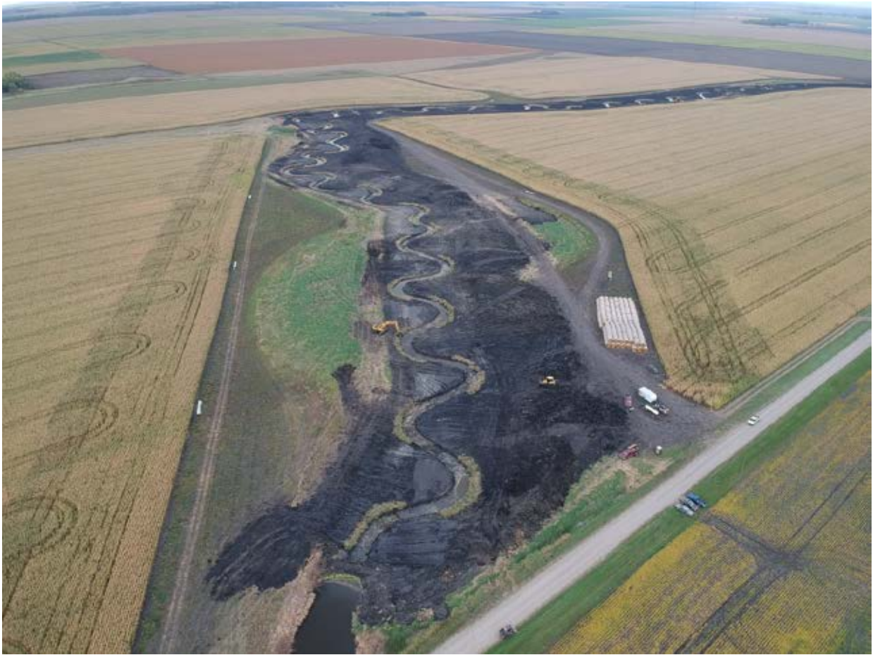
Photo 13-7. Aerial view during construction. Photo provided by the BRRWD.
