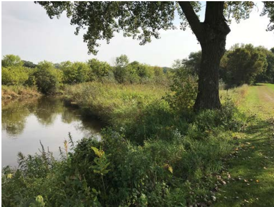
Photo 32-3 View of a lowered point bar to create a wetland terrace that is fully vegetated making it appear at almost the same elevation as the surrounding landscape. (Wedge Creek – Reach 6, photo taken by Lucius Jonett during site visit 09/20/2019).
