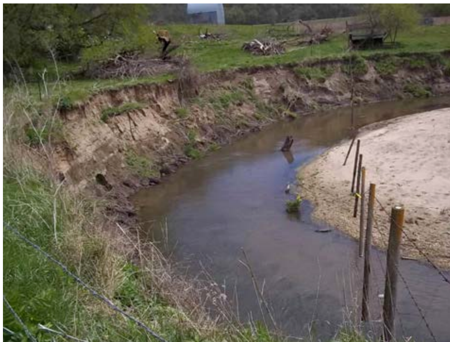
Photo 29-3 Example of an eroding bank taken in 2011 prior to the construction project. Photo provided by John Lenczewski, MNTU.
