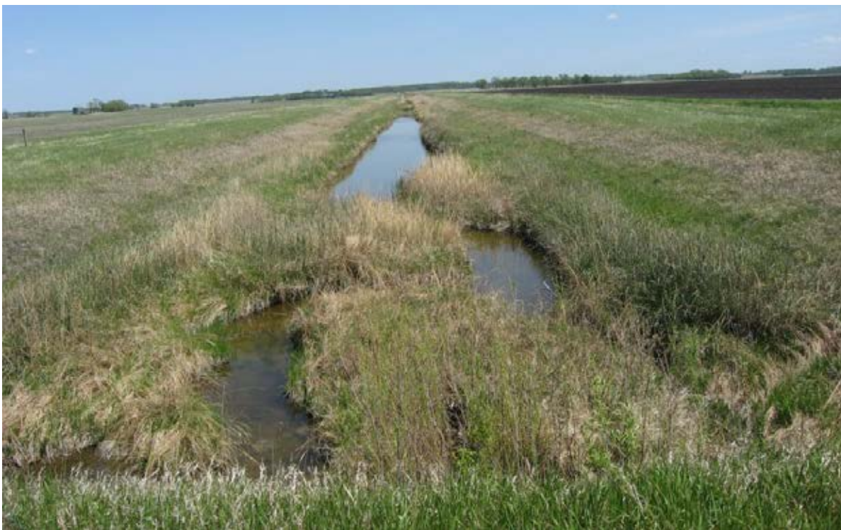
Photo 14-1 Burnham Creek pre construction and channel cleanout. Photo taken by project partners (5/2/2012).
