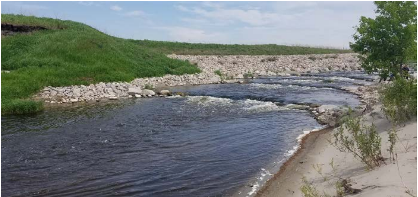
Photo 16-8 Sand Hill River fishway ramp #2 after the original drop structure was modified for fish passage. Volunteer sandbar willow is establishing on the right bank. Photo taken by Ed Matthiesen during site visit (6/4/2019).
