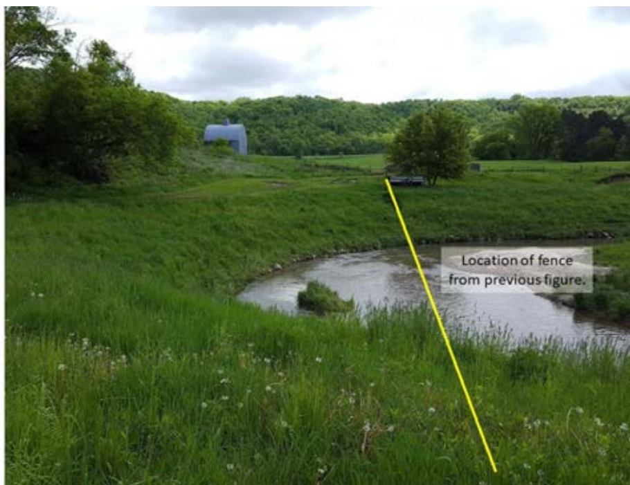
Photo 29-4 Example of the same bank as Photo 29-1 in July 2019, 8 years after the project was completed. Photo provided by John Lenczewski, MNTU.
