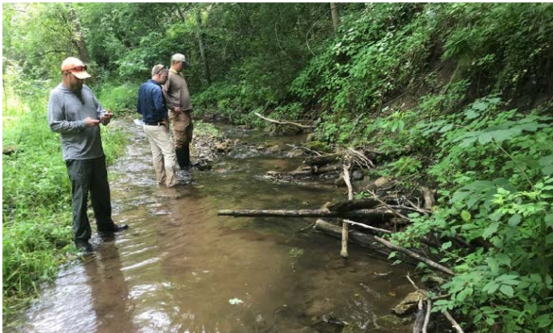
Photo 39-4 Photograph of Toewood Stabilization (right side of photo) constructed by hand labor. Structure has degraded substantially in 4 to 5 years since installation but is still provide some habitat and stability benefit. Photograph taken by Kevin Biehn during 7/18/2019 site visit.
