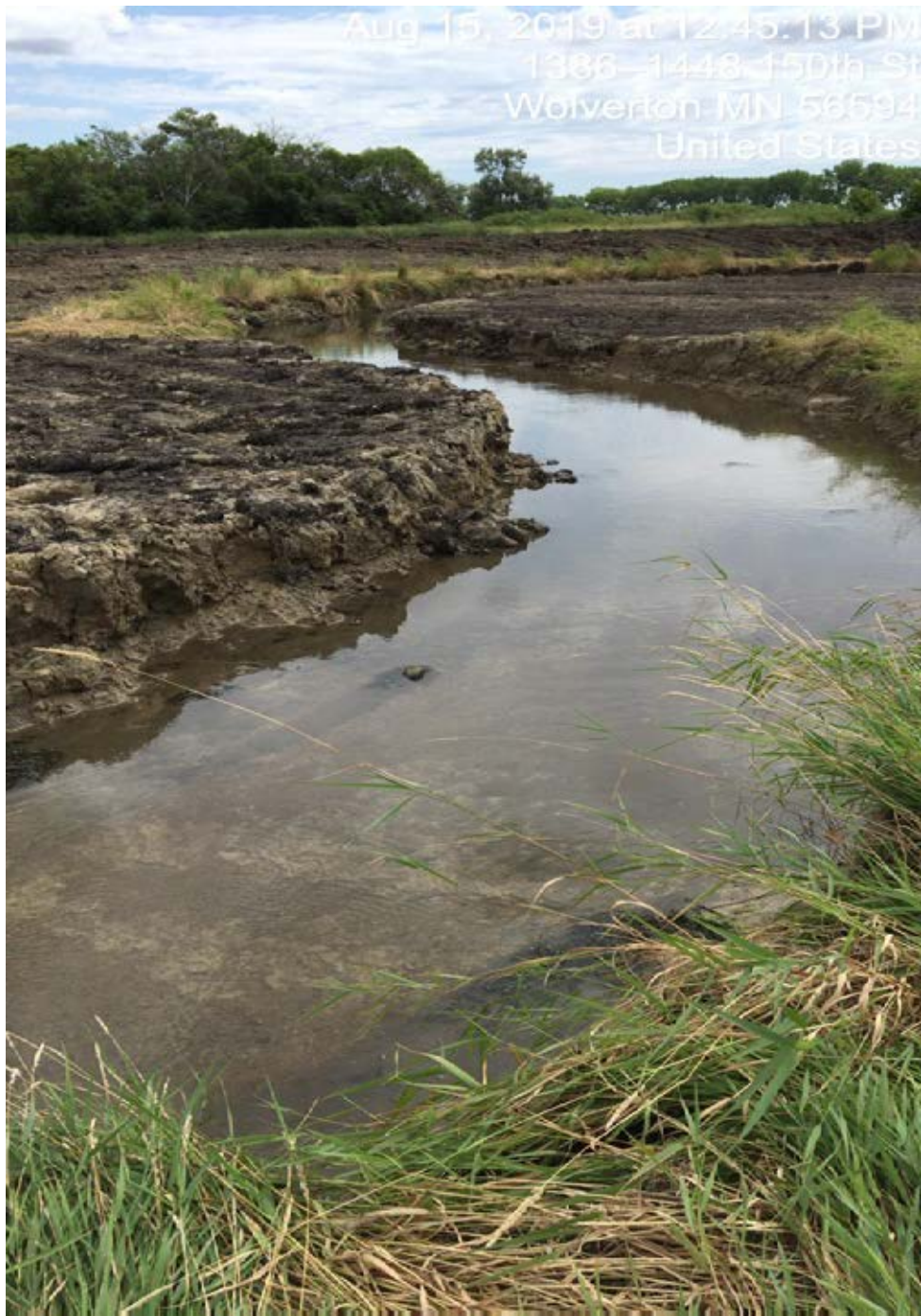
Photo 13-3. Recently constructed channel showing reed canary sod mats and two-stage Rosgen E channel design. Photo taken by Anna Varian during site visit (8/15/2019).
