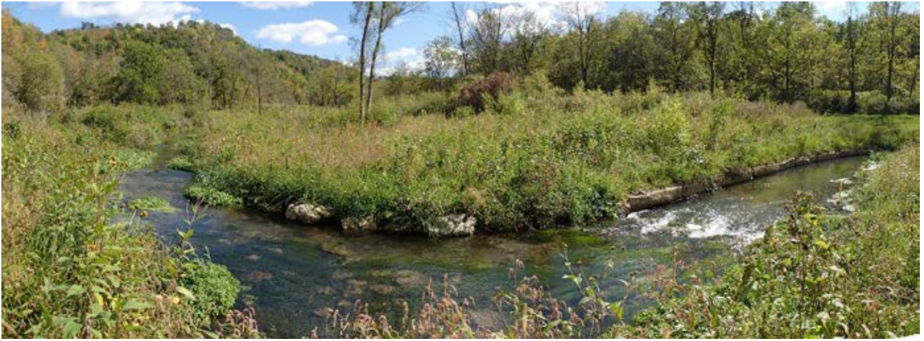
Photo 33-9 Panoramic photo of reconstructed stream bend with rock weir and rip rap and sky hook on opposite streambank. Site visit 09/18/2012.
