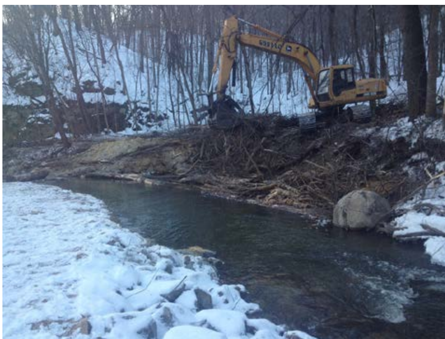
Photo 31-4 Cribwall during construction. (Seven Mile Creek County Park, December 2016).
