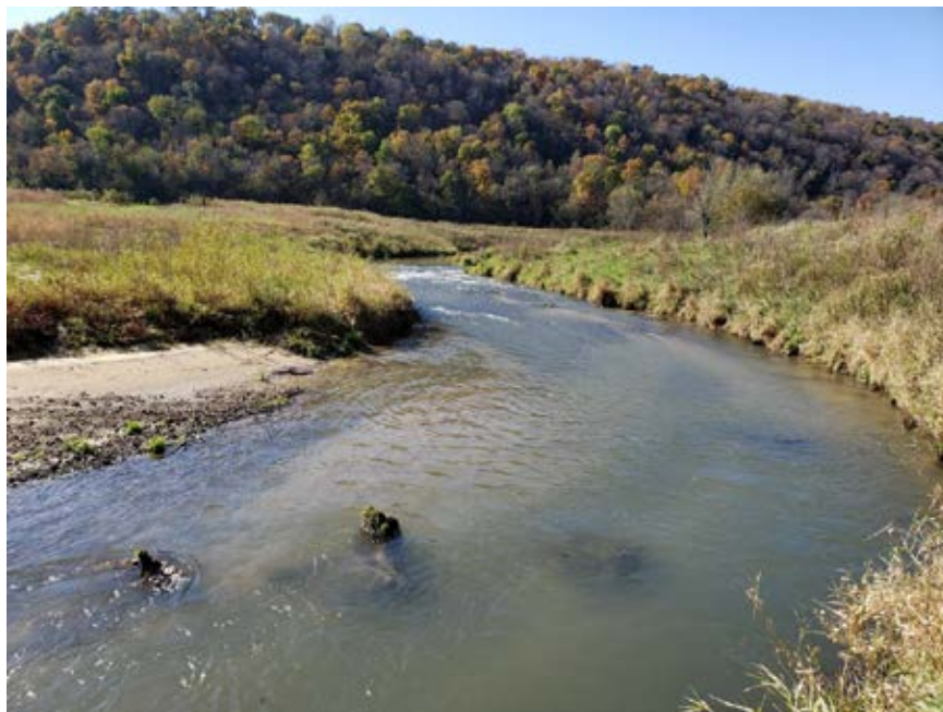
Photo 29-6. Example looking upstream near the middle of the project reach. Random boulder cluster in the foreground. A J-hook with a designated cattle crossing where riffles are occurring. Photo taken on 10/18/19 by Mark Pranckus, Cardno.
