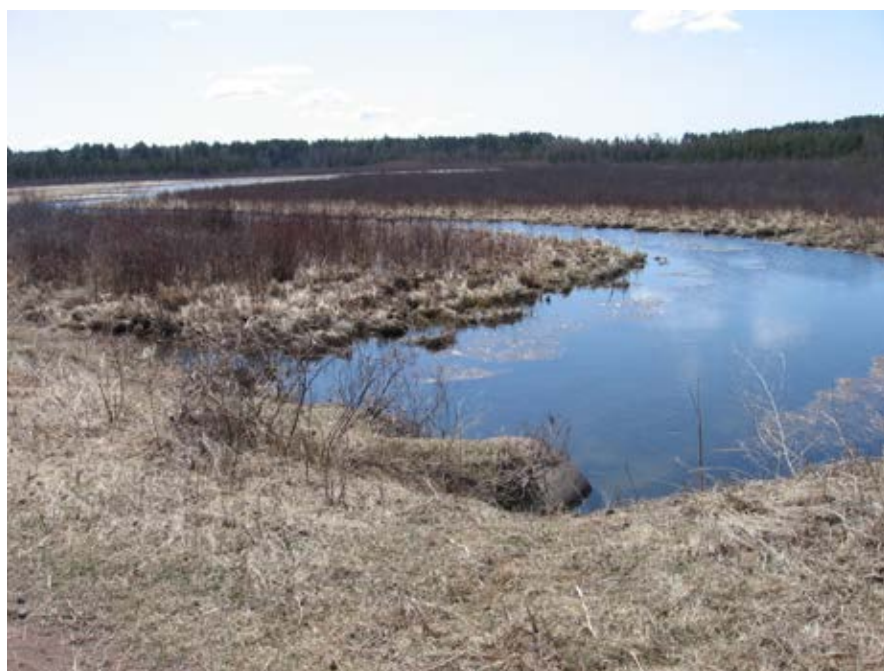
Photo 23-2 Downstream view from the Portage Lake dam prior to removal.
