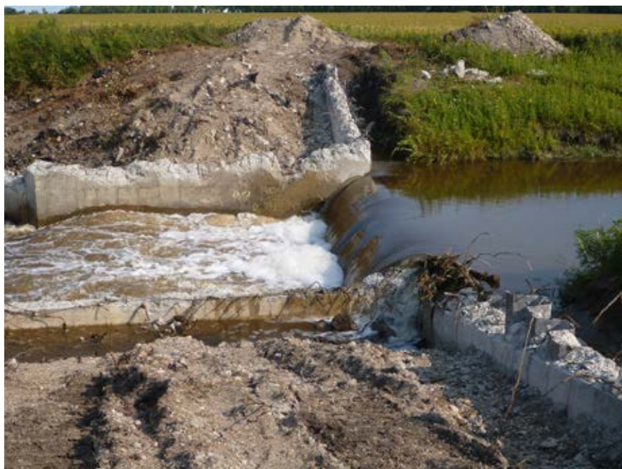
Photo 16-2 Drop structure 4 during removal. Photo provide by project partners (taken 9/1/2016).
