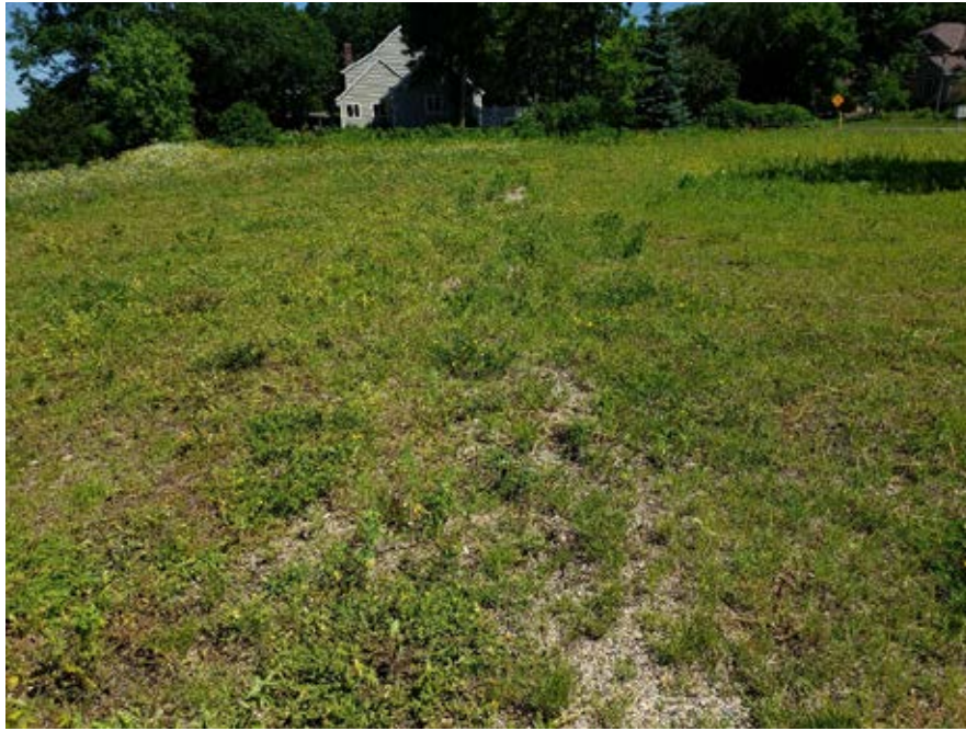
Photo 30-9. Example of the native vegetation seeded at the top of the slope to control surface water. Water flowing on the surface during storm events is ponded and captured in the French drain and is routed via drain tile to the base of the slope. (Photo taken 6/26/19 by Mark Pranckus, Cardno).
