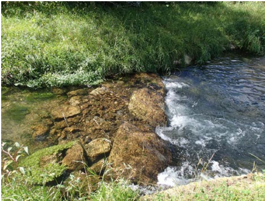
Photo 33-6 Rock weir structure. Site visit 09/18/2012.
