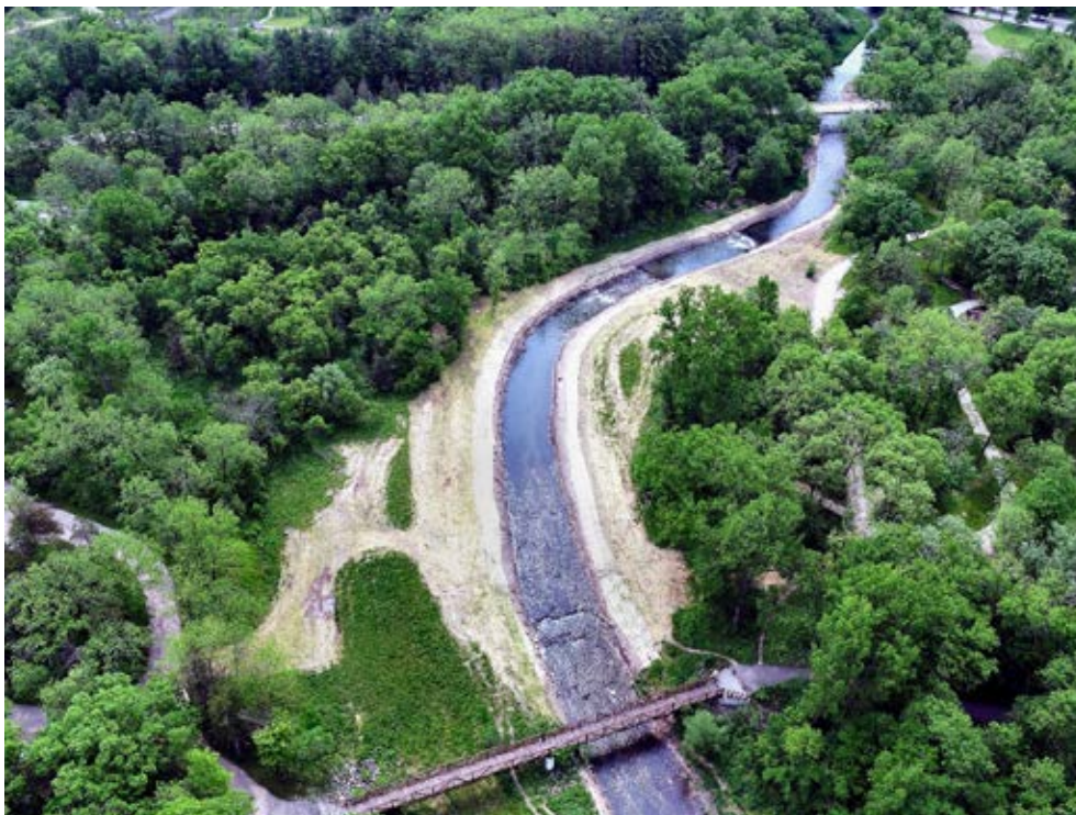
Photo 36-4 Aerial view of project site taken after project construction in early summer 2019.
