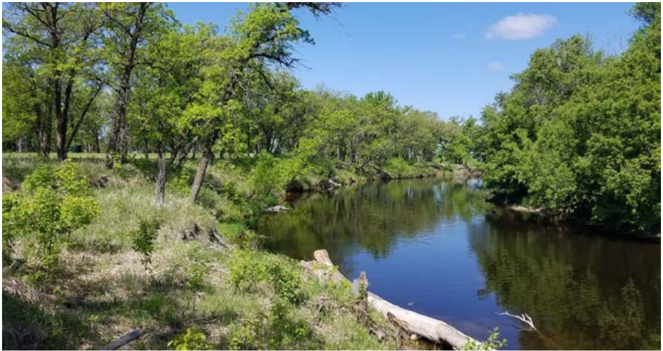
Photo 11-3 Upstream view of stream barbs 6, 7, and 8. Photo taken by Ed Matthiesen during site visit (6/5/2019).
