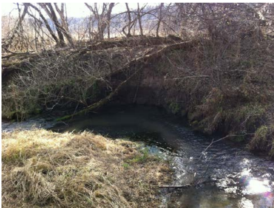
Photo 19-1 Pre-project conditions, photo taken in November 2012.
