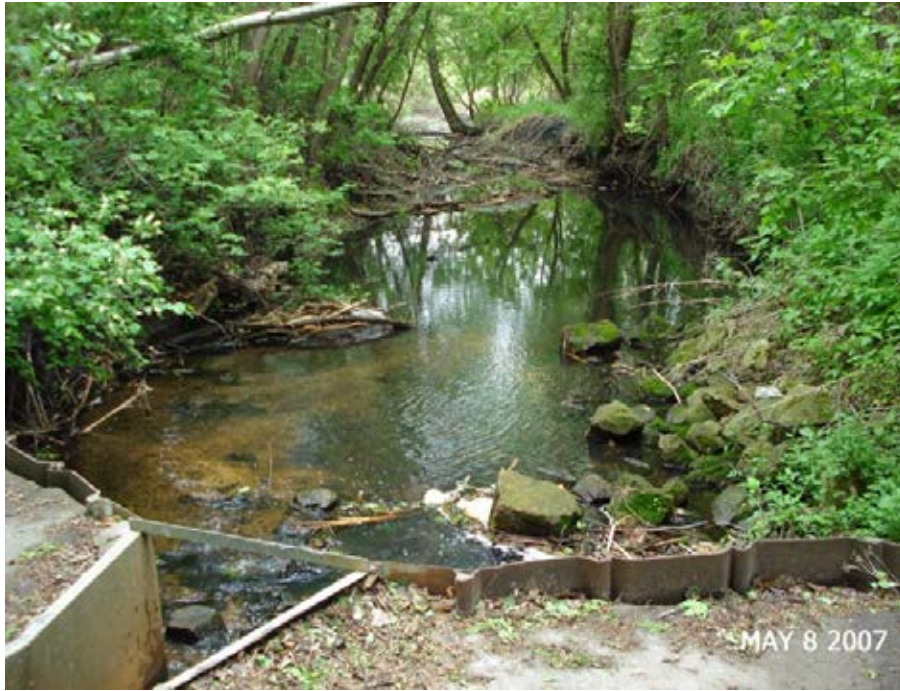
Photo 7-1 Before project image immediately downstream (west) of existing flume. Photograph provided by VLAWMO, dated May 8 2007.
