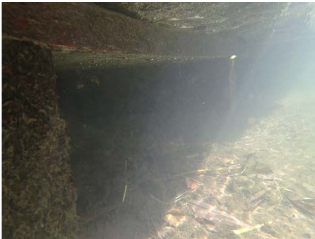
Photo 33-8 Underwater support for Sky-hook structure shown in Photo 33-7. Site visit 09/18/2012.
